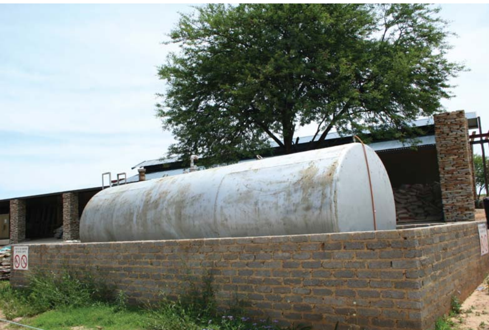
Bunding around the temporary diesel tank to guard against spillage can hold one and a half times the volume of the tank.
