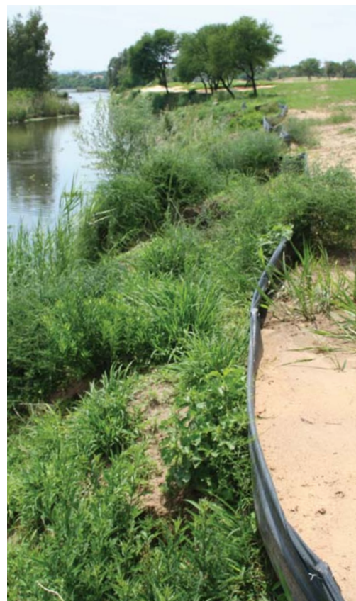
BELOW LEFT and BELOW: The entire Vaal de Grace site is encompassed by silt fences. Claudia Holgate standing astride the fence demonstrates the silt build-up on the side away from the river, after the recent rains.
